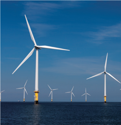
SIEMENS transformer in wind power.
